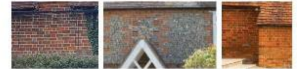
Flemish bond with contrasting headers. Decorative brickwork detailing quins/ dressings. Flint in-fill. Handmade facing brickwork - red / orange.
