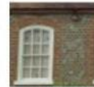
Decorative brickwork detailing, quoins/dressings
