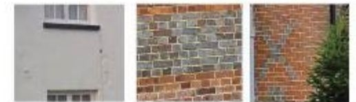
Painted render. English bond. Contrasting brickwork bands. Decorative brickwork.
