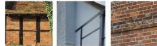
Timber frame with brick infill
