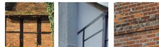
Timber frame with brick infill
