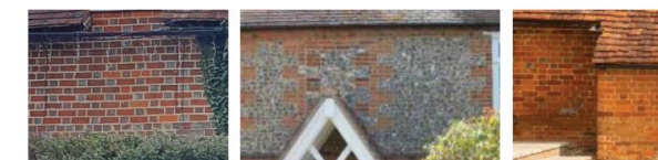
Flemish bond with contrasting headers
