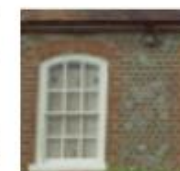
Decorative brickwork detailing, quoins/ dressings
