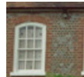
Decorative brickwork detailing, quoins/ dressings
