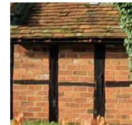
Timber frame with brick infill
