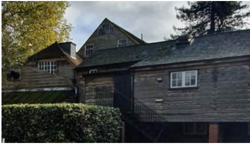
Sonning Mill - Grade II Listed
