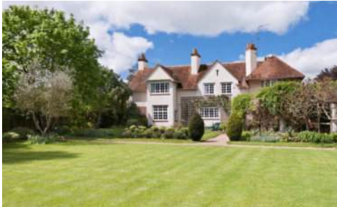
Eyot House - Grade II* Listed
