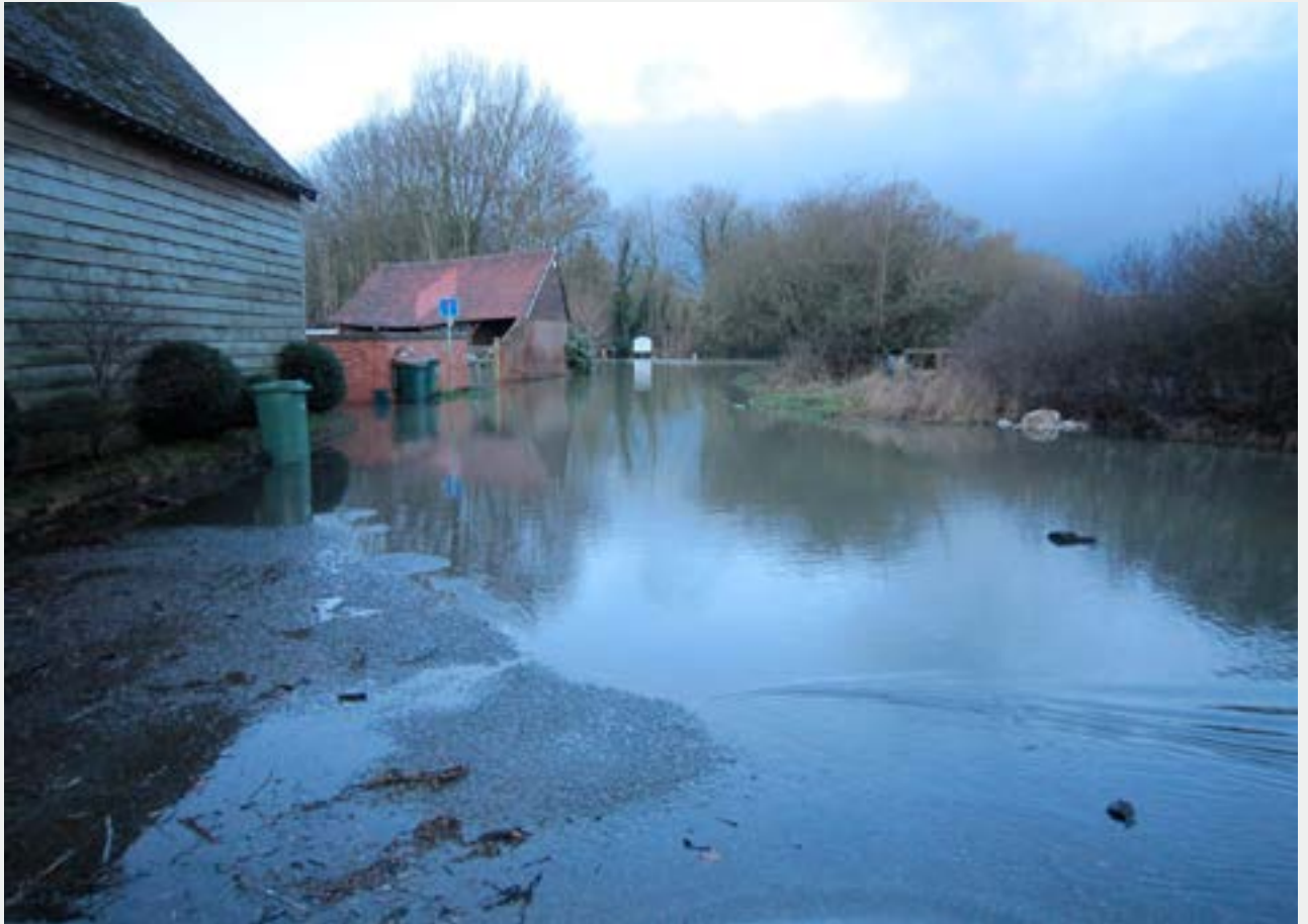
■ Old B478 Flooding, 2009
