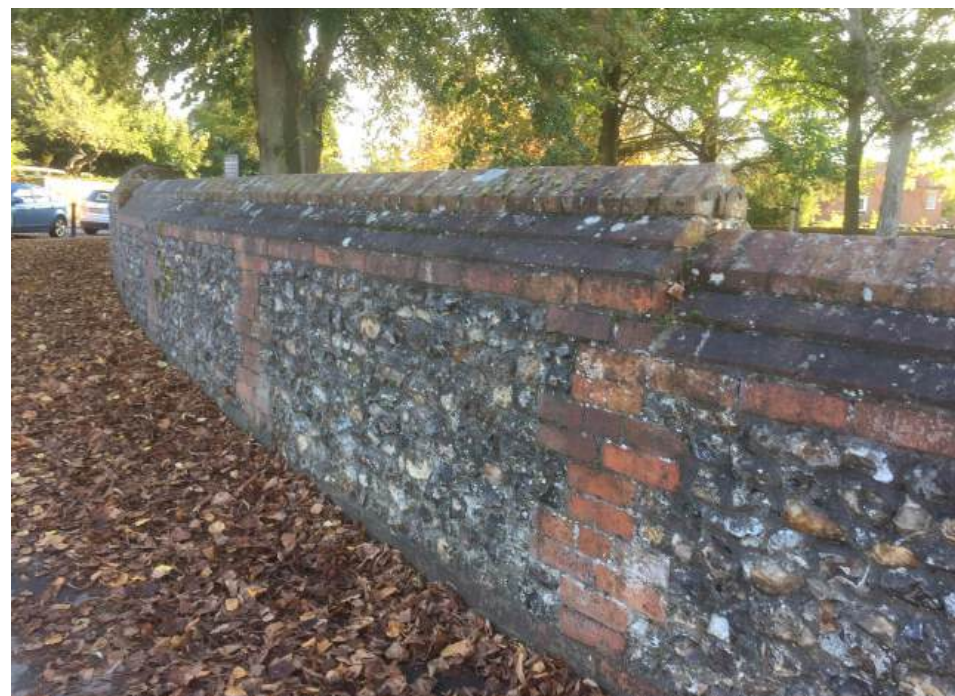
Fig 51. Rectory Garden brick and flint wall
