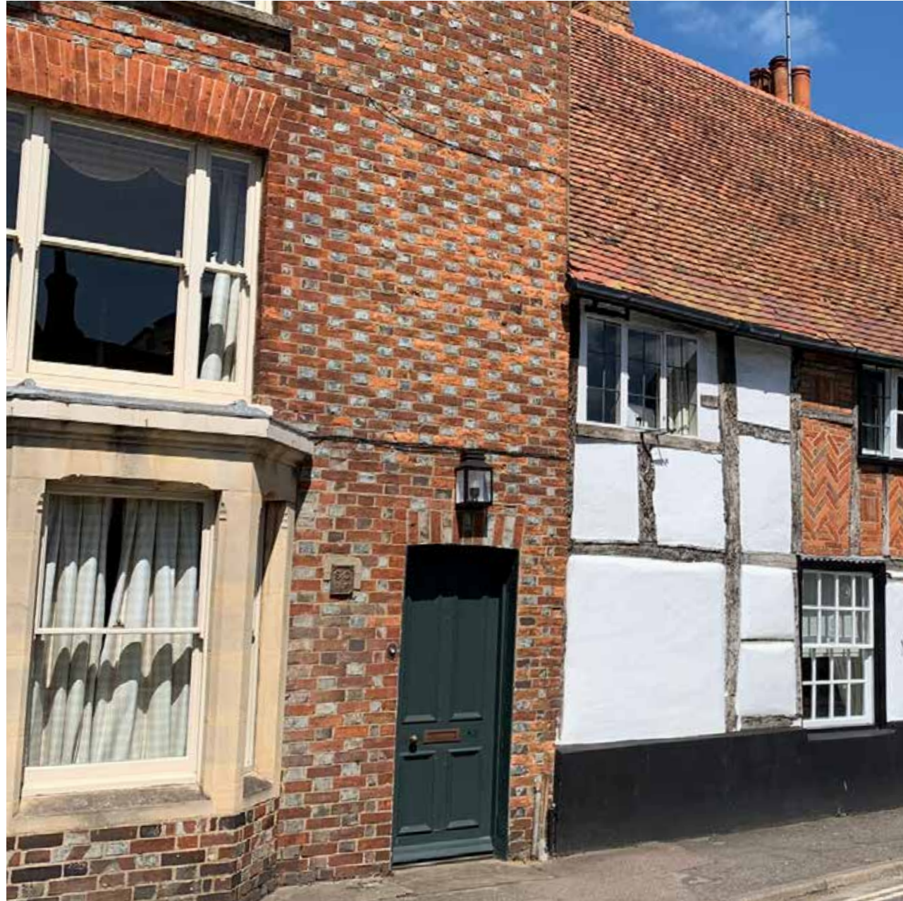
Figure 48: Use of contrasting brick pattern to create decorative interest
