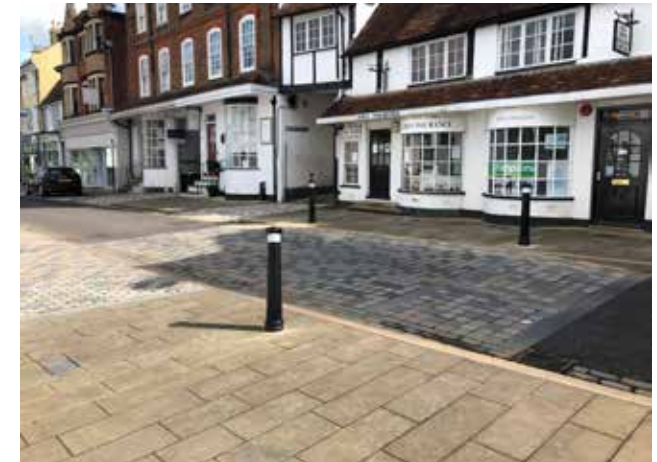
Figure 88: An example of raised pedestrian crossing with a plateau in Hemel Hempstead
