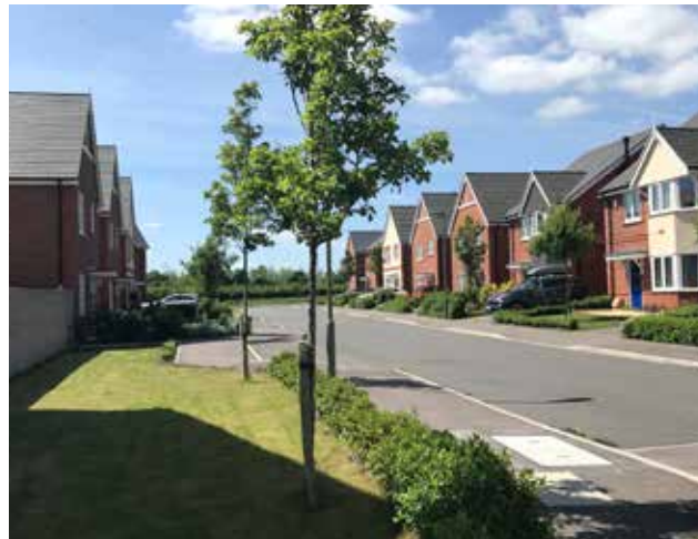
Figure 150: Well defined private space to front
