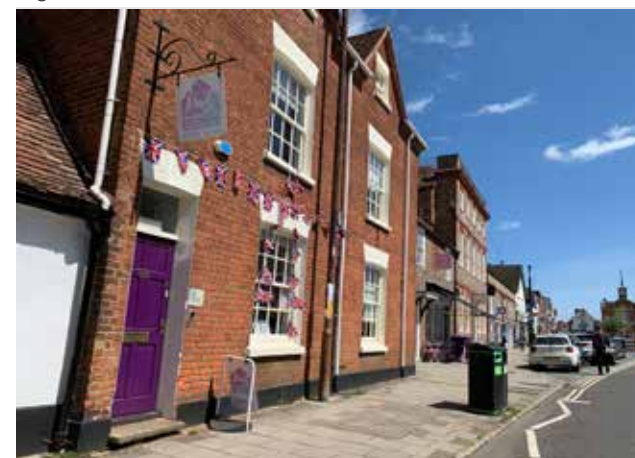
Figure 143: Consistent building line with no set back or protruding features in the town centre - CA1
