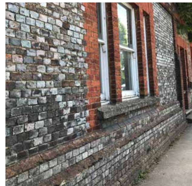
Figure 44: Use of contrasting brick to accentuate window openings
