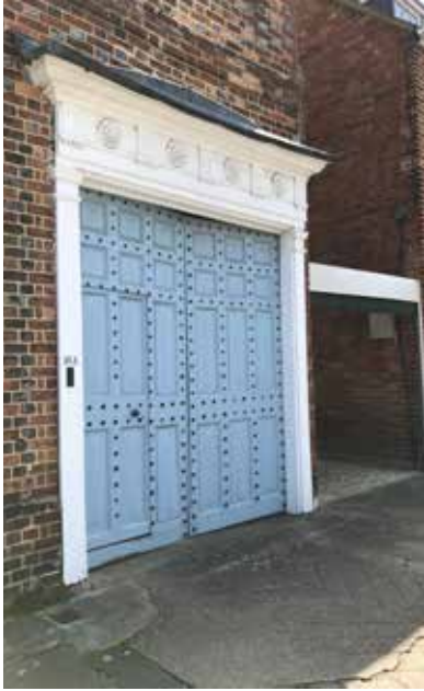
Figure 45: Feature door, Upper High St
