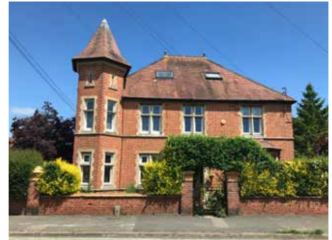
Figure 09: Example of grand Victorian manor house, with typical red brick finish and stone window casing
