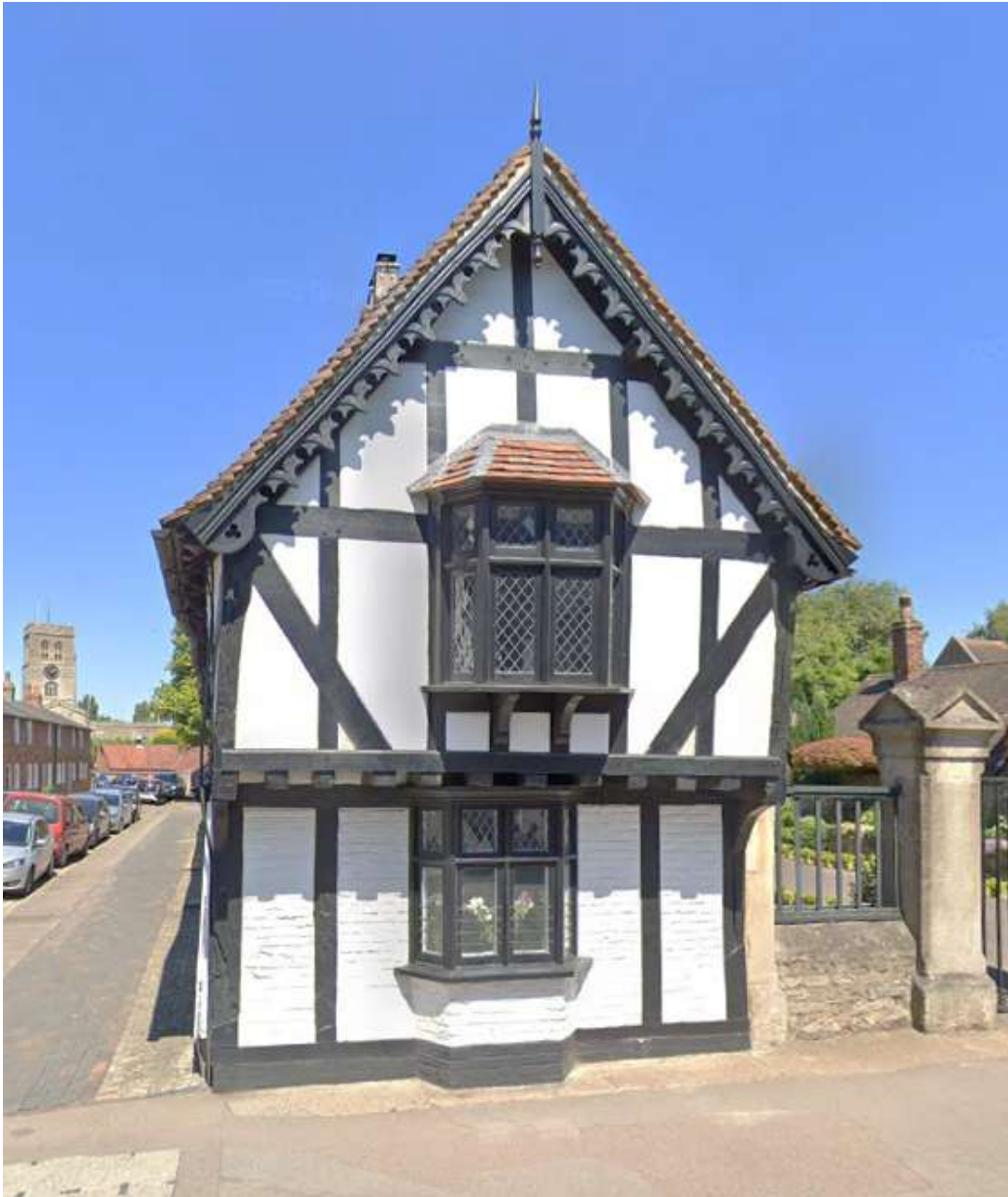
Figure 11: Several buildings are of timber-frame design and construction (Source: Google StreetView)
