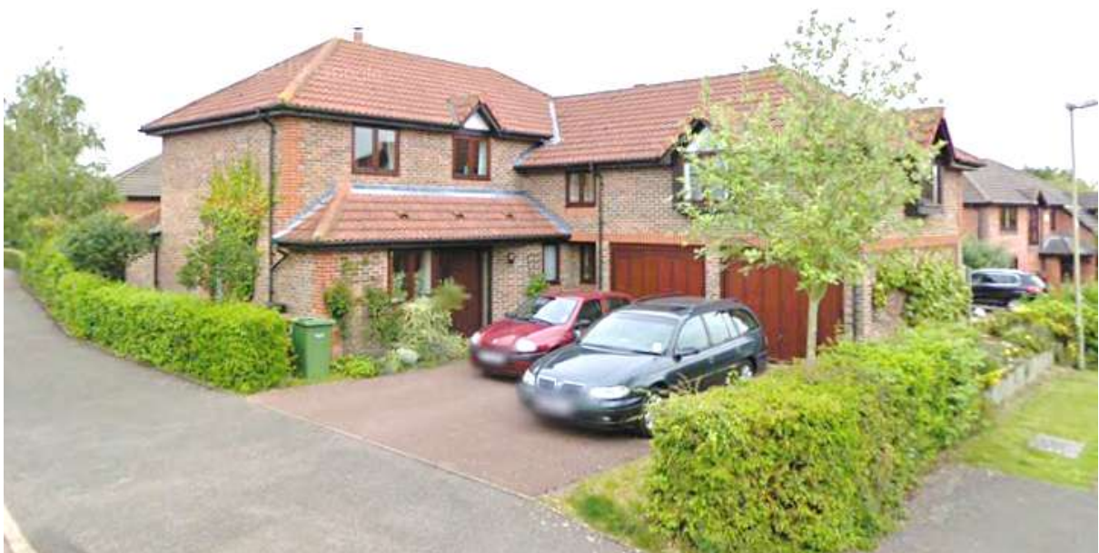
Figure 32: Properties along Maple Road are more modern, and in general larger than the original properties in the adjacent streets (Source: Google StreetView)
