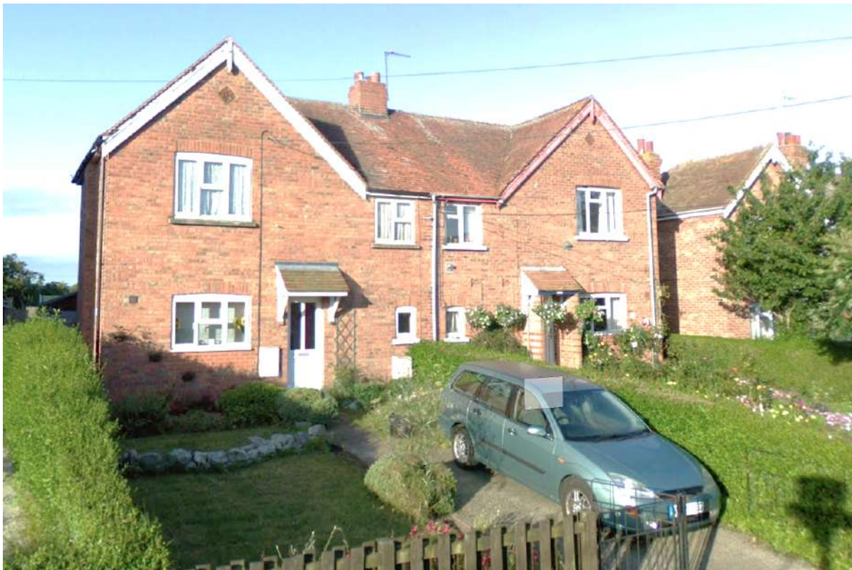
Figure 22: Semi-detached properties on Hampden Avenue (Source: Google StreetView)
