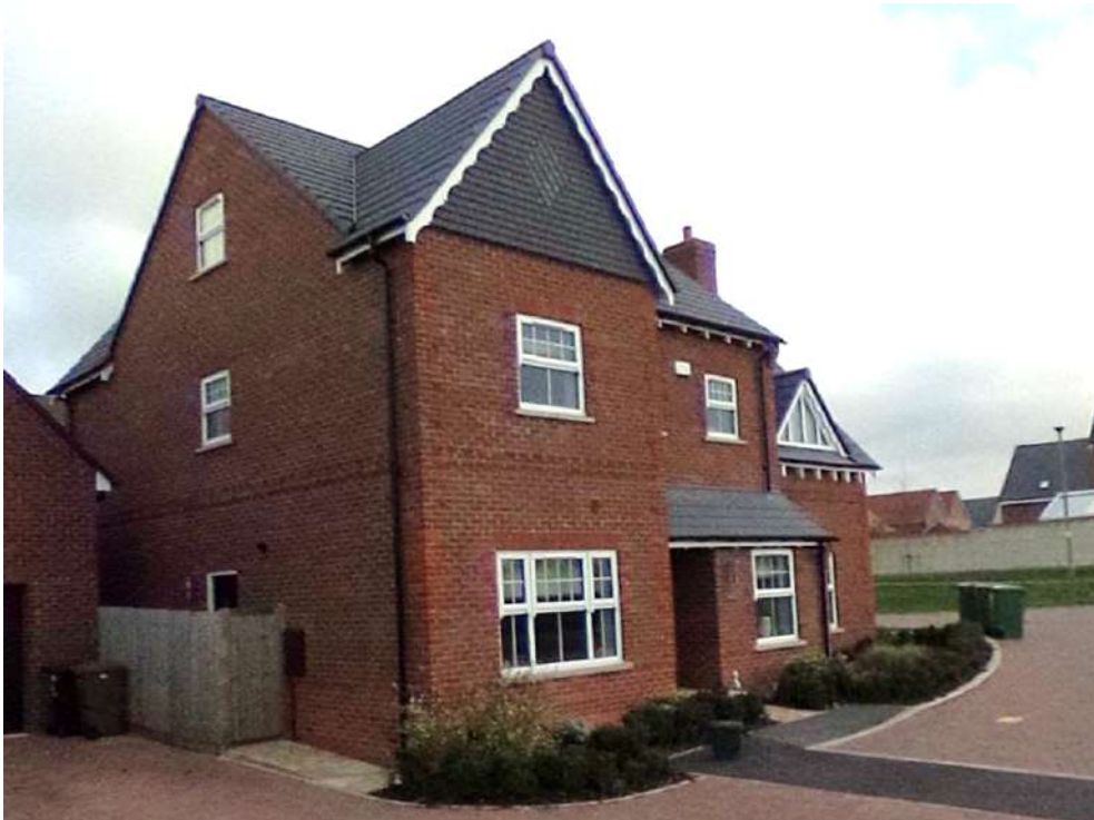
Figure 51: Large family home featuring a cross gabled roof and small front garden such as the one pictured are common in the area (Source: Google StreetView)
