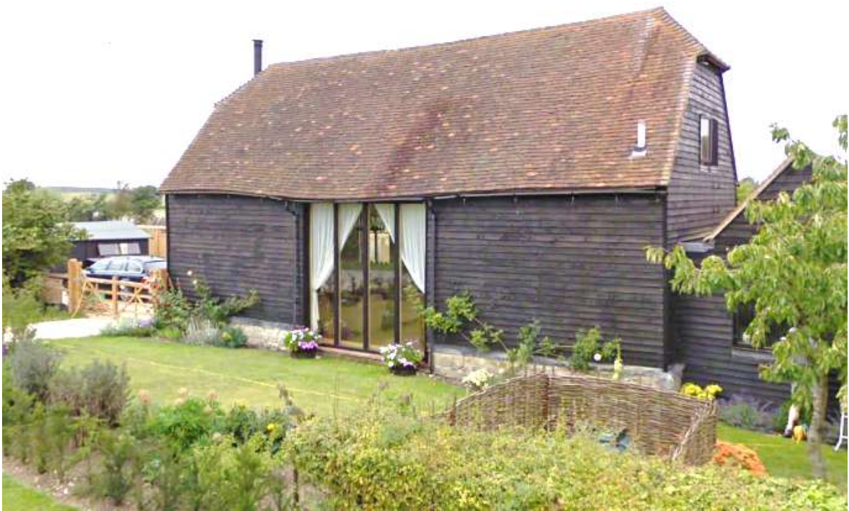
Figure 37: Converted barn with a half-hipped roof (Source: Google StreetView)
