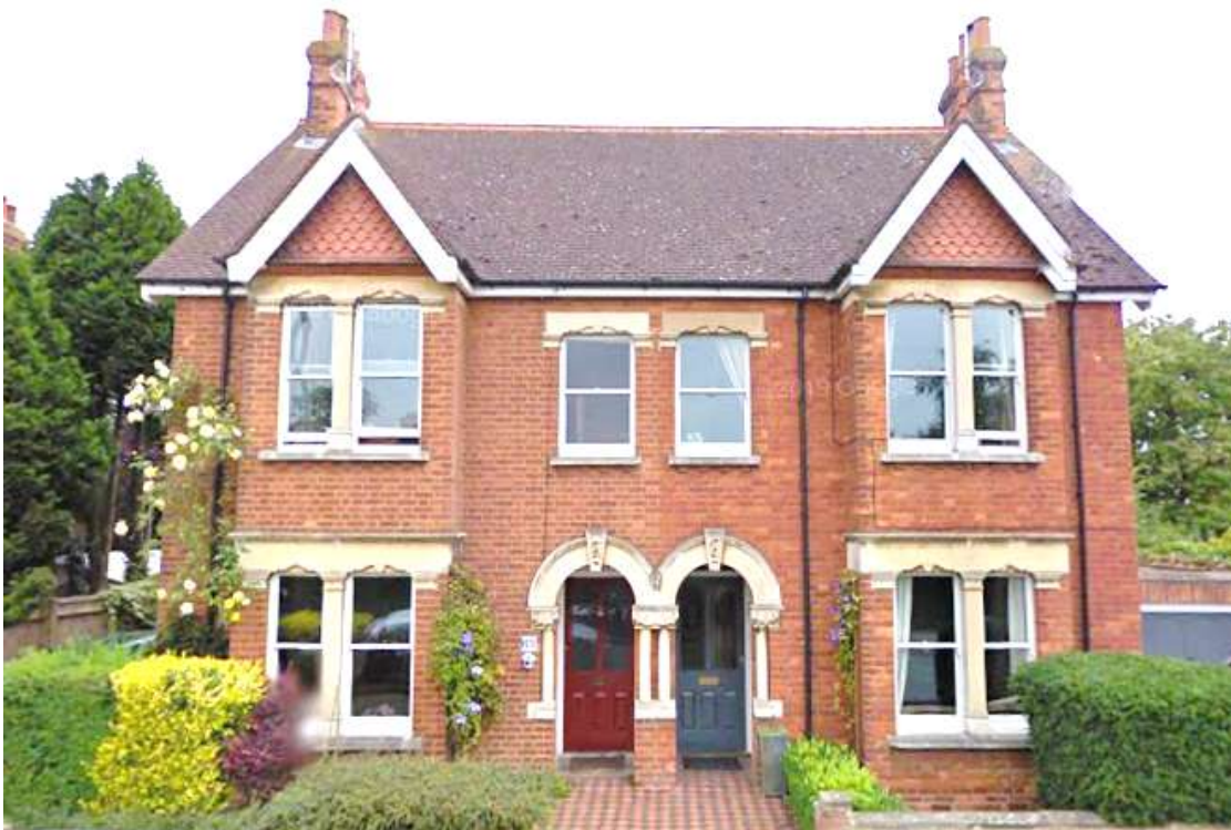
Figure 43: Victorian style houses, with small front gardens and decorative arches (Source: Google StreetView)
