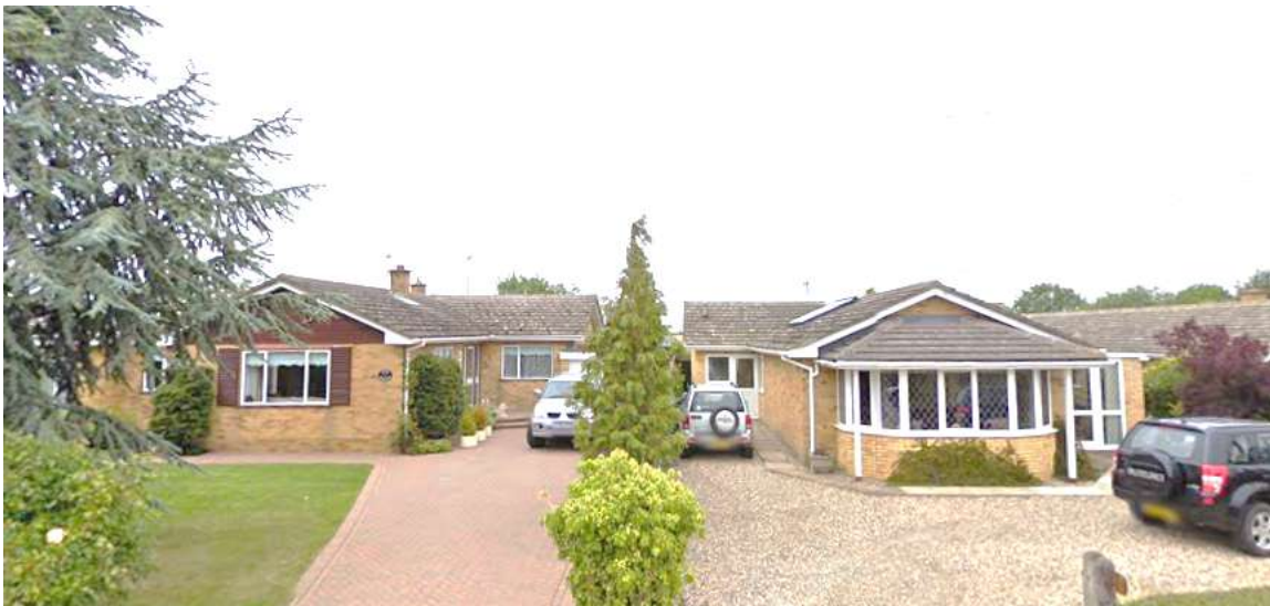
Figure 35: Bungalows with large front gardens, both have off-street parking (Source: Google StreetView)
