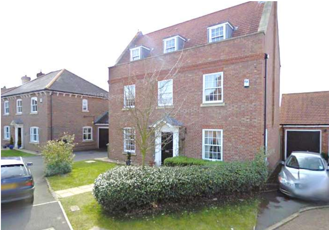
Figure 44: New build homes made from brick, often making use of the roof space, providing three storeys of accommodation but responding to the prevailing two-storey height of the majority of properties in the area. (Source: Google StreetView)
