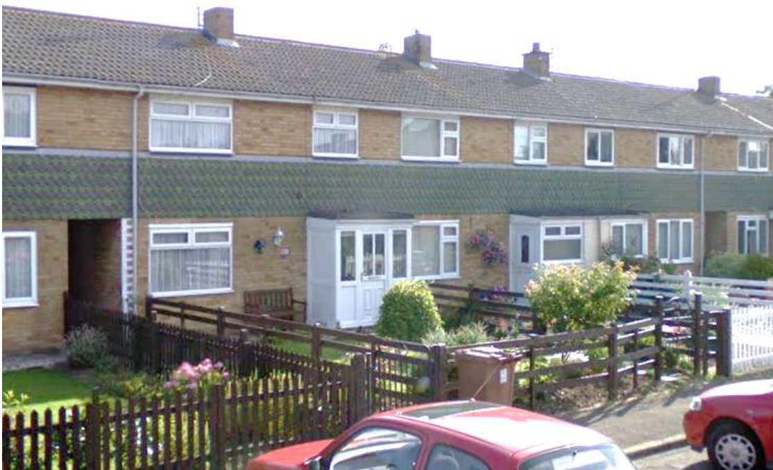
Figure 45: Terraced properties constructed using brick and weatherboarding and have enclosed front gardens. (Source: Google StreetView)
