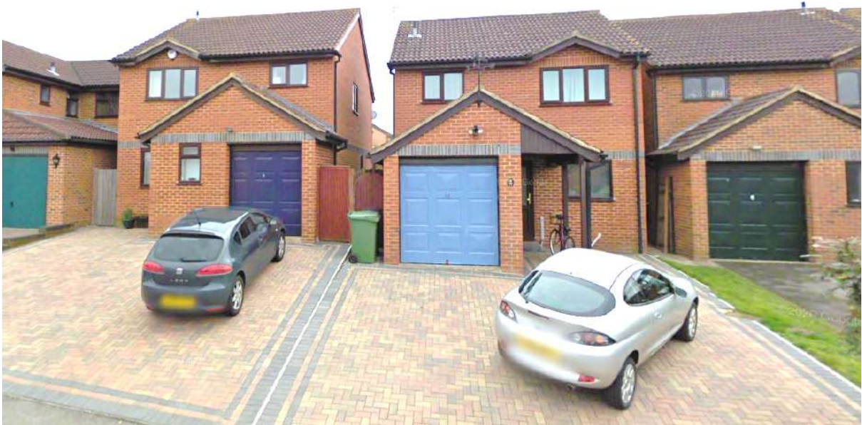
Figure 16: There are many two-storey detached brick properties where front gardens have been paved over to provide off-street parking (Source: Google StreetView)
