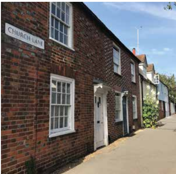
C18 vitrified header brickwork, Church Lane
