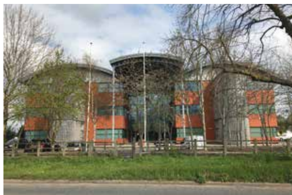
Former Habitat showroom and warehouse
