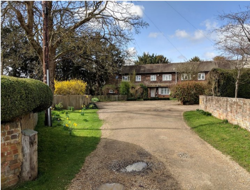
Picture 1: The Old Barn Cottages from the High Street
