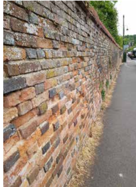
Fig 66. Deteriorating masonry wall, High St
